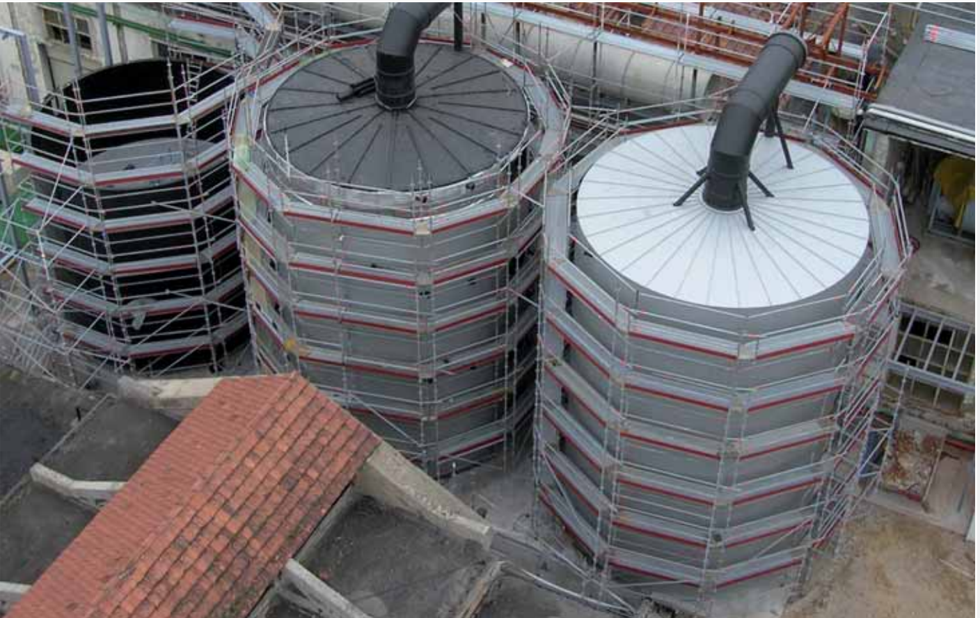
13 meter high silos was made of HDPE, Spain (Photo: Colasit)
