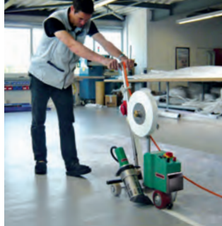
Welding tapes at maximum speed.
