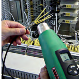
Shrinking of cable labels
