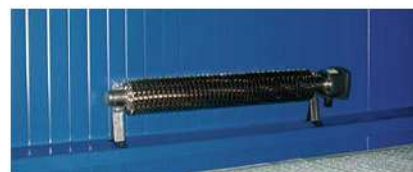
Installed example of ribbed pipe heating
