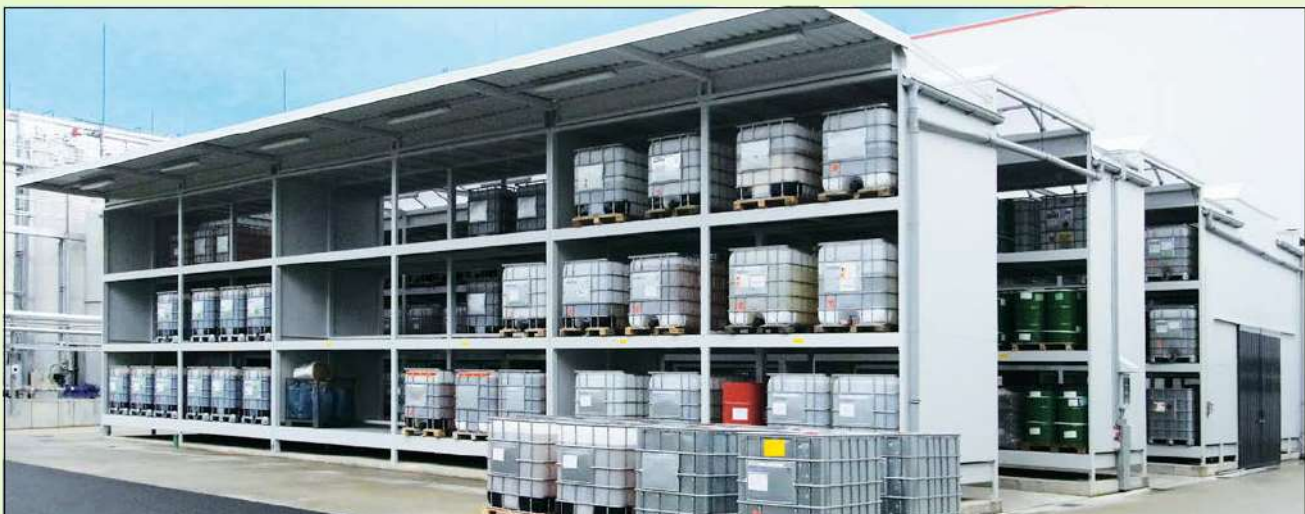
Large scale store for approx 400 tonnes of hazardous materials in drums, IBC / ASF and other special containers, fully covered, with efficient access to each container
