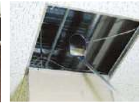
For inspection in ceiling
