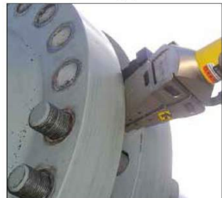
▼ Flange maintenance and joint separation with FSH-14 Hydraulic Wedge Spreader.
