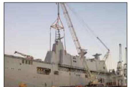
Synchronous hoisting and load positioning
