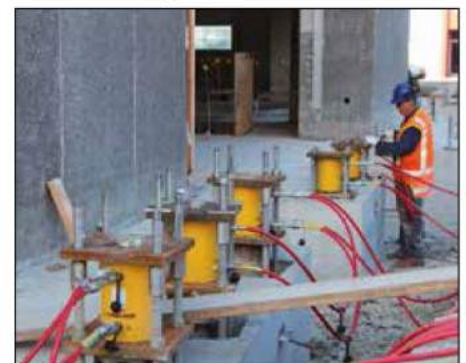
▼ Foundation repair: Synchronous lift system used to lift a 1000 ton building.
