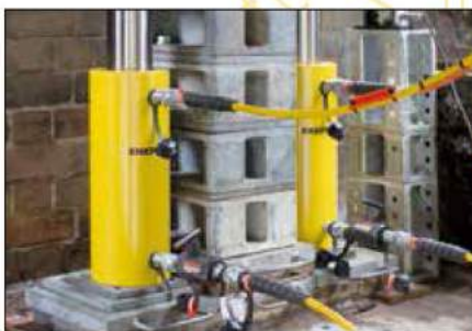
Bridge lifting and launching
