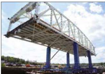
Incremental bridge lifting
