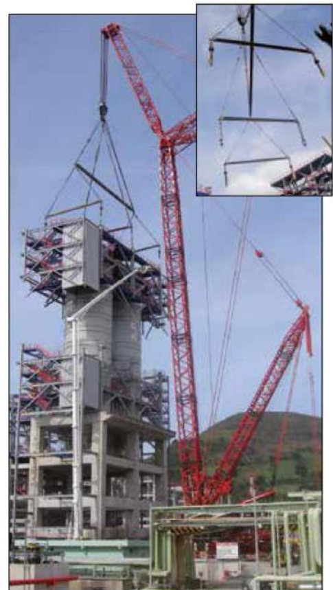
SyncHoist system mounted in an auxiliary frame for levelling and positioning steel structures during construction of an oil & gas installation. ▶
