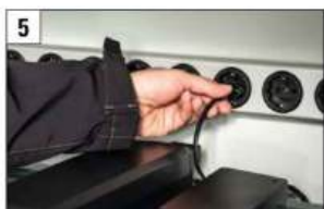
5 Socket board with metal housing and protected sockets
