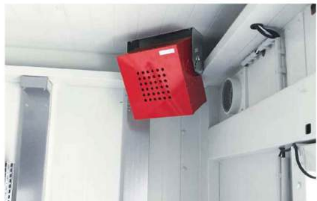
The aerosol extinguishing system is triggered by temperature and effectively interrupts the chemical combustion process within 4.5 - 15 seconds (depending on model).
