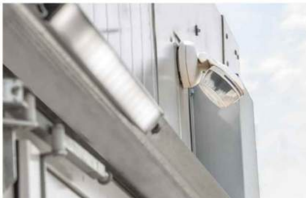
External lighting with motion sensor.
