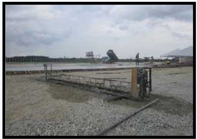
Vibratory Trusses Screed
